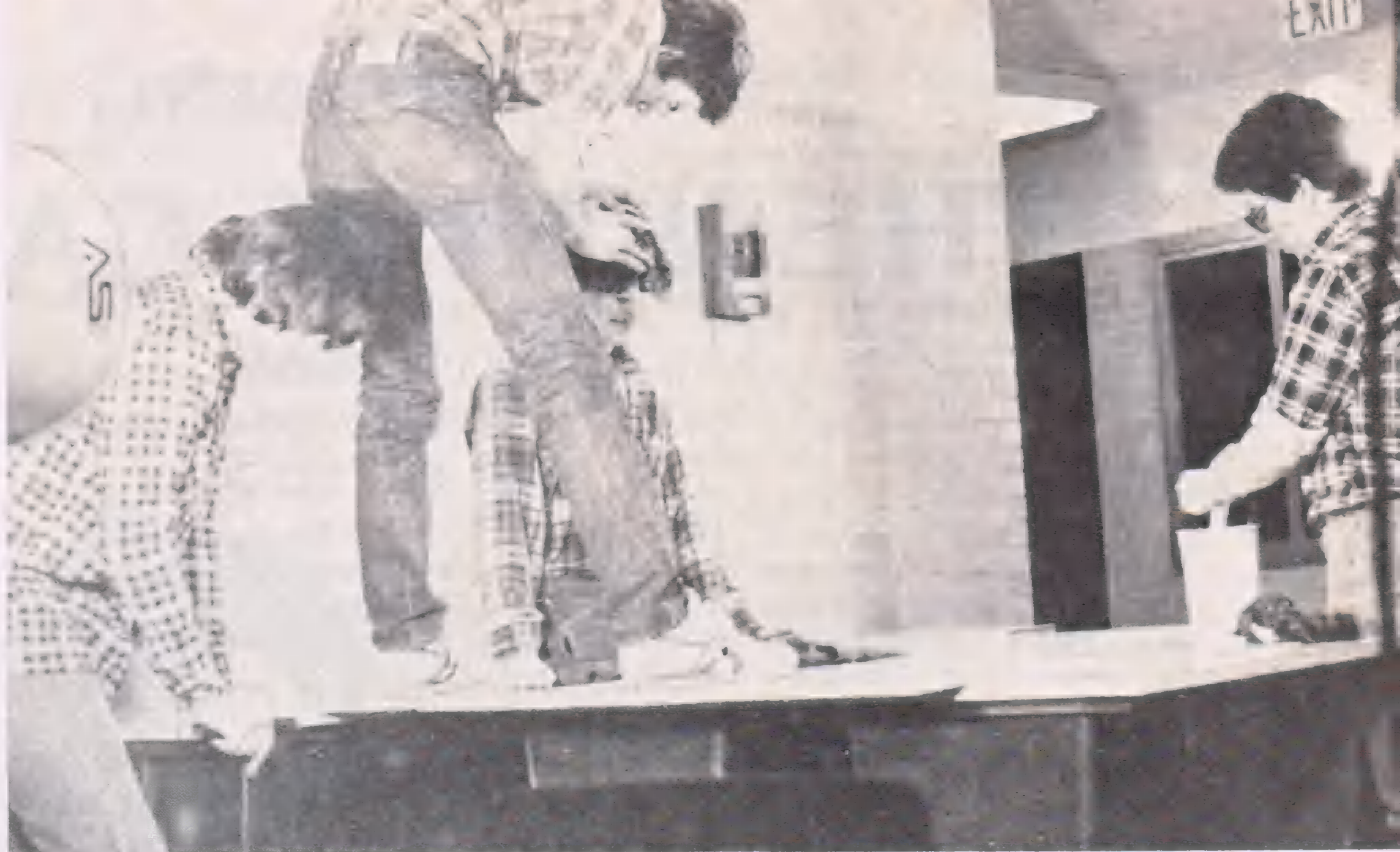
A behind-the-scenes look at the false floor that was constructed for North Hills High School's production, A Witch in Time . The floor was mounted on tables so actor Richard Huebner could slide beneath it.
